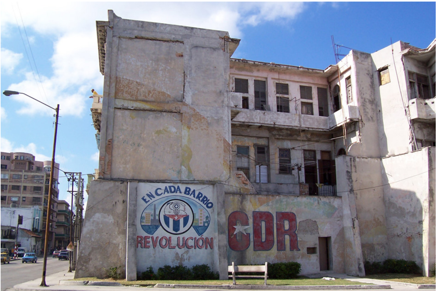
Figure 1: "In every neighborhood, Revolution! Dilapidated building in Central Havana, Photo by Author, 2004.
